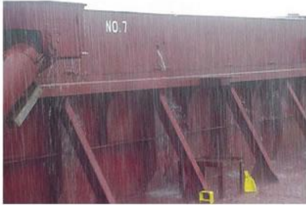
Hose testing and ultrasonic hatch testing for leaks
