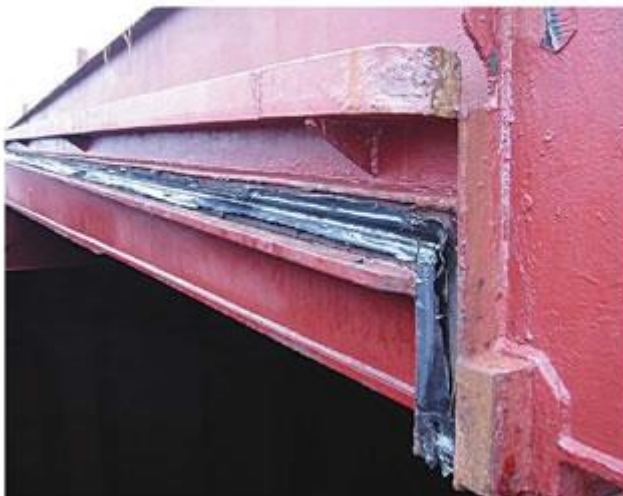
Poor practice: hatch tape used to build up cross joints. This is discouraged
