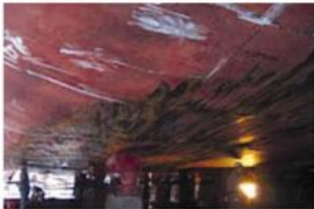
Lack of awareness of surrounding dangers led to significant hull damage for this container ship. Photo: MAIB
