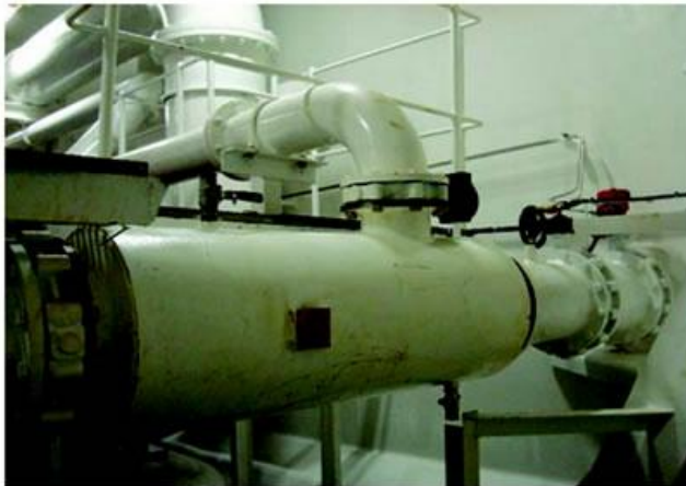
GSA Marine's Swirl Absorber seen fitted on board Navion Hispania.
