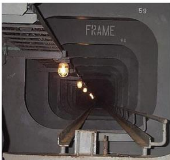
Void space in inner bottom.
