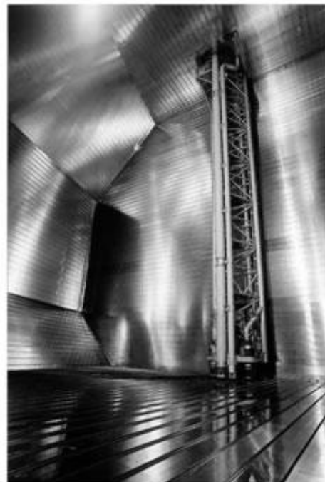
Fig. 12 View of interior of completed cargo tank
